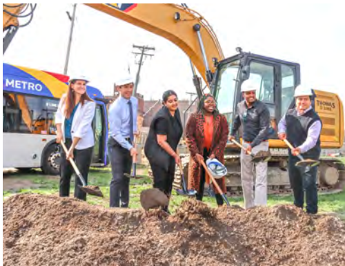
Ground broke in 2022 for the Bus Rapid Transit B Line. It will link Uptown in Minneapolis via Lake Street to downtown St. Paul via Marshall and Selby.
